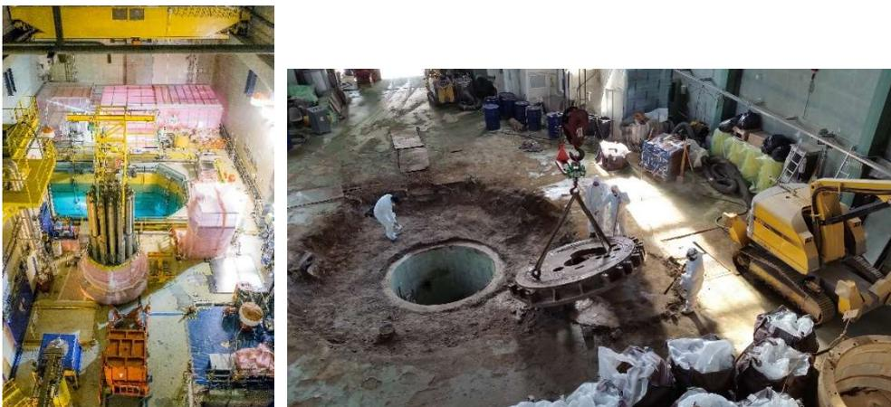
FIG. A-4. Dismantling of Chooz A nuclear power reactor components, France (left), and decommissioning progress at the Magurele research reactor, Romania (right). (Photos: EDF, IAEA)
